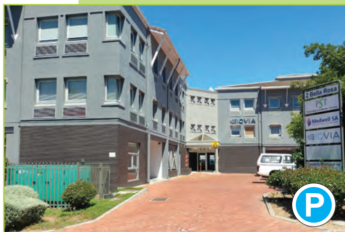
MONTROSE PLACE: MAIN ENTRANCE
