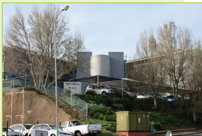
MONTROSE PLACE: VIEW FROM DURBAN ROAD
